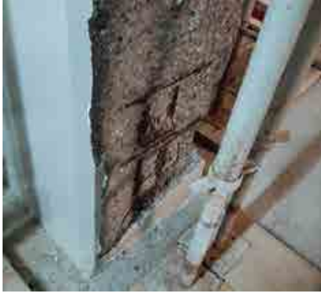
The inevitable end result of all rebar corrosion is concrete damage.
